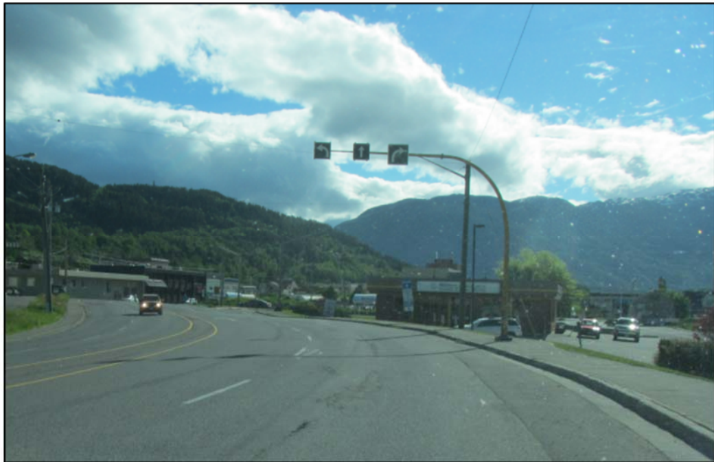
Figure 28: Arterial Road Example – Greig Avenue
