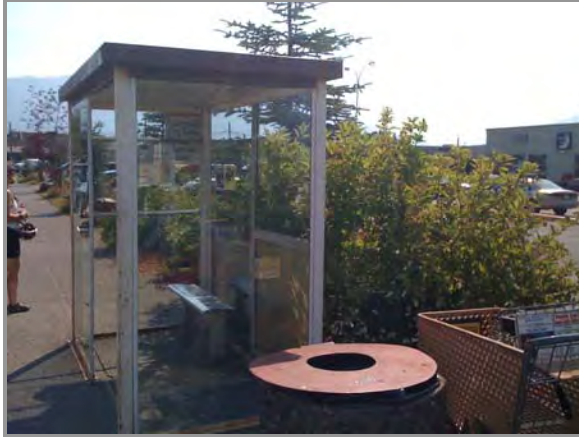
Figure 21. Transit stop with shelter, bench and posted schedules
