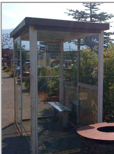
Bus shelter with amenities
