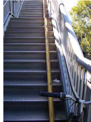
Staircases retrofitted with wheel gutter feature
