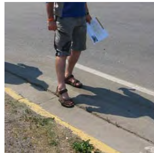
Pavement to gutter transition on Sparks St. Photo: H.Redman
