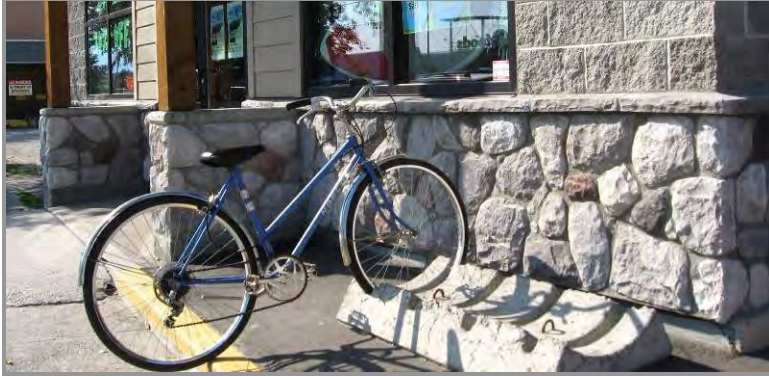
Figure 5. Wheel-bender bicycle rack
