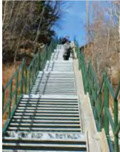
Staircases built with ramp for bicycles
