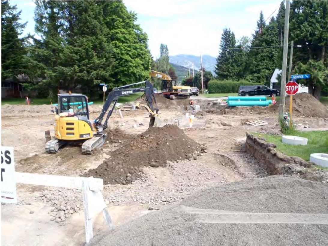
Figure 31: Munroe Street Road Construction Project
