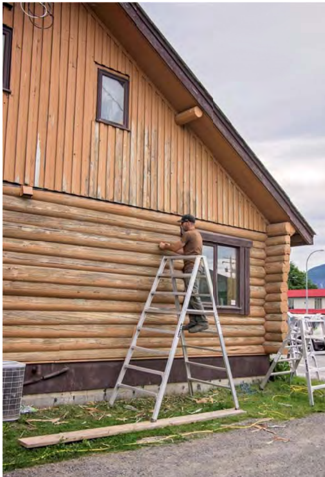
Figure 29: Work on the Visitor Information Centre
