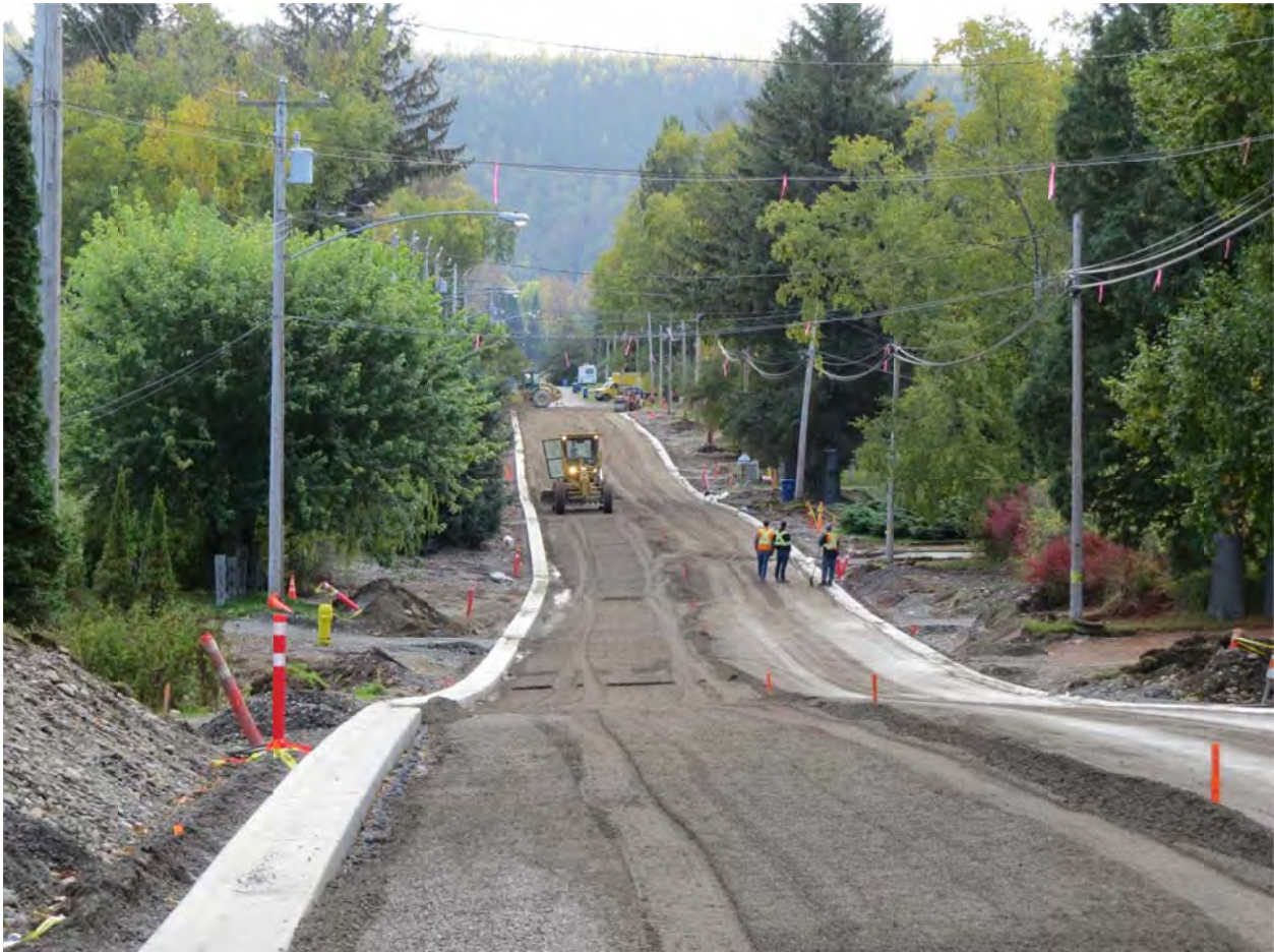
Figure 30: Kalum Street Road Construction Project
