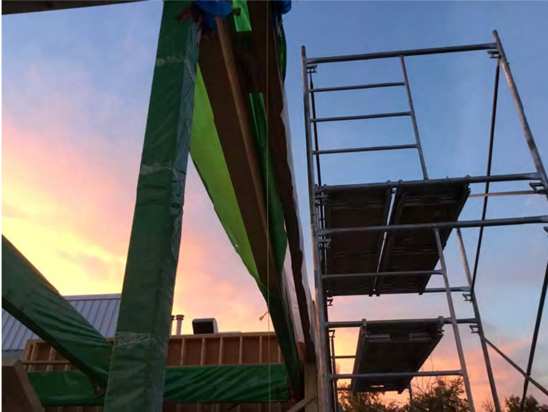
Figure 25: Scaffolding at the Terrace and District Aquatic Centre
