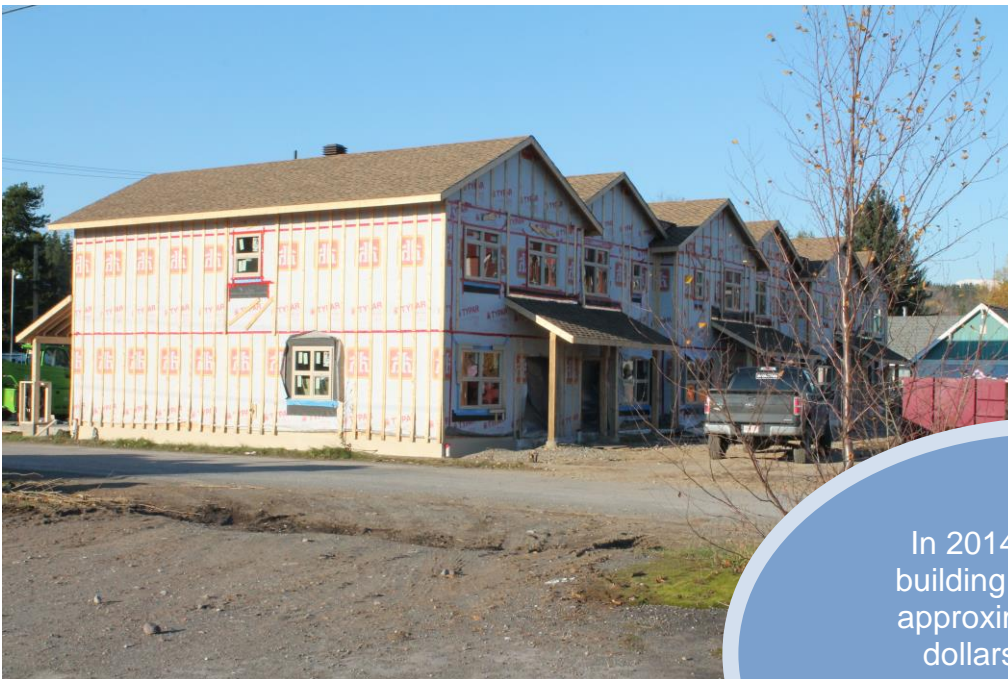
New housing development in Terrace.
