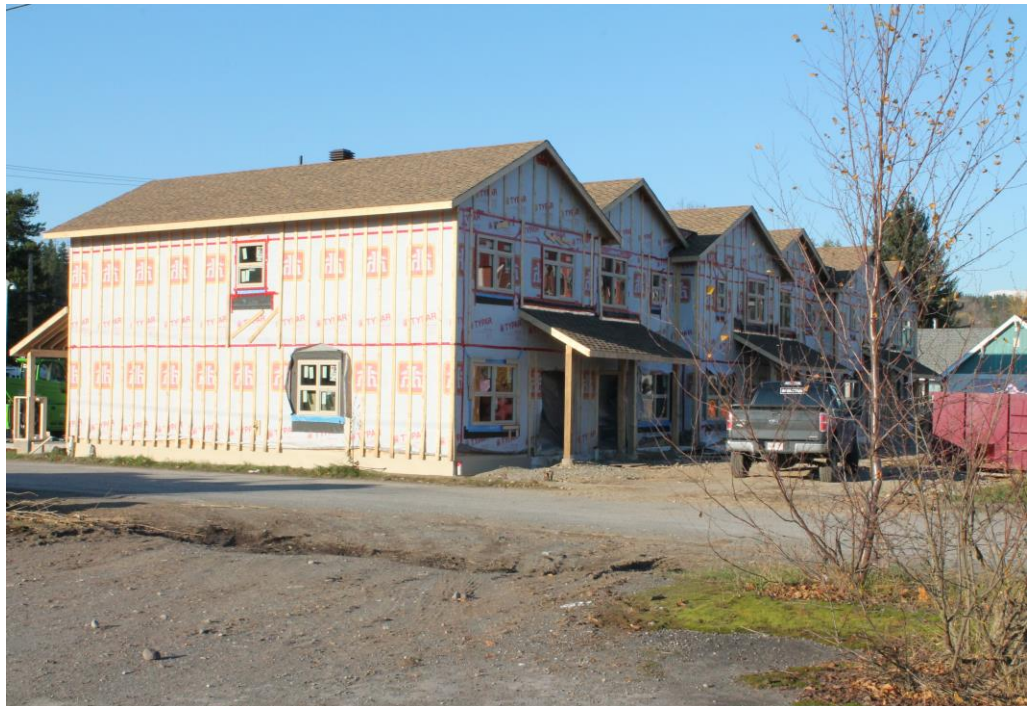
Development of multi-family housing in Terrace.
