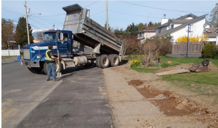
Post-construction rehabilitation of residential areas.
