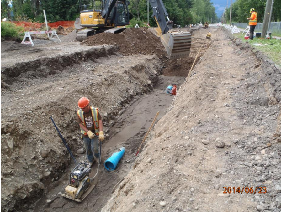
Infrastructure work on Graham Avenue.
