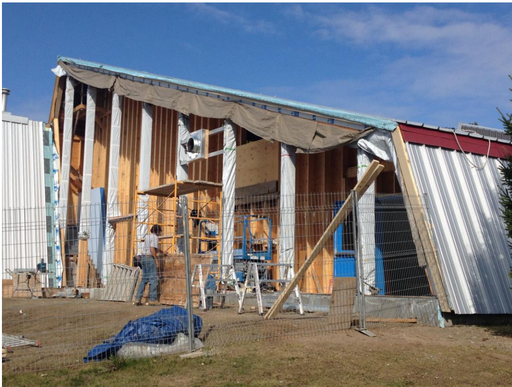
Terrace Aquatic Centre renovations.
