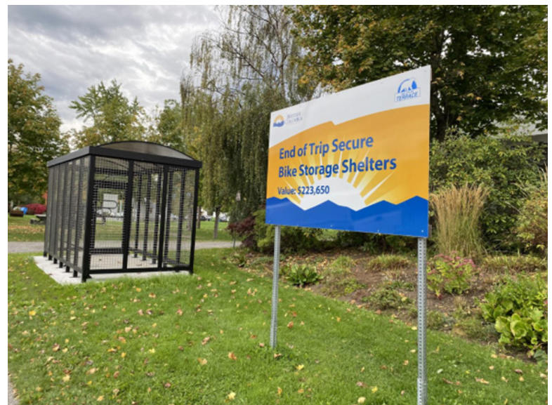
Above: Bike Shelter installed outside the Terrace & District Public Library
