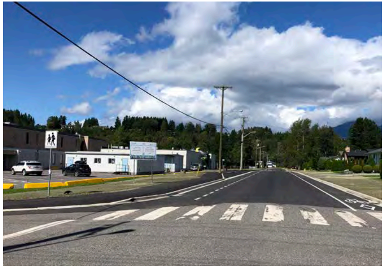
Above: In 2020, Public Works crews completed road reconstruction on Munroe Street from Straume Avenue to McConnell Avenue, at a cost of $1 million.
