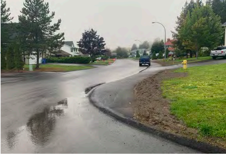
Left: In 2020, Public Works crews completed road reconstruction in the 5200 block of Mountain Vista Road.
