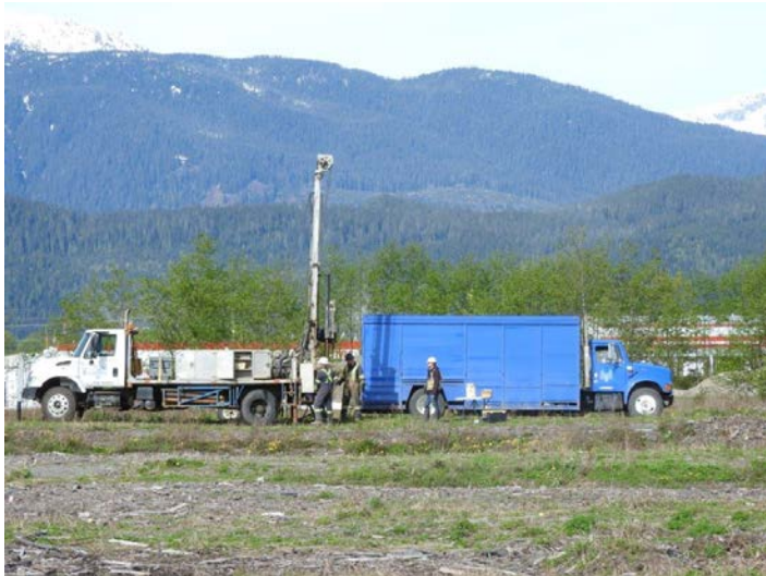
Well drilling to monitor water and soil at the City owned Keith/Kenney property.
