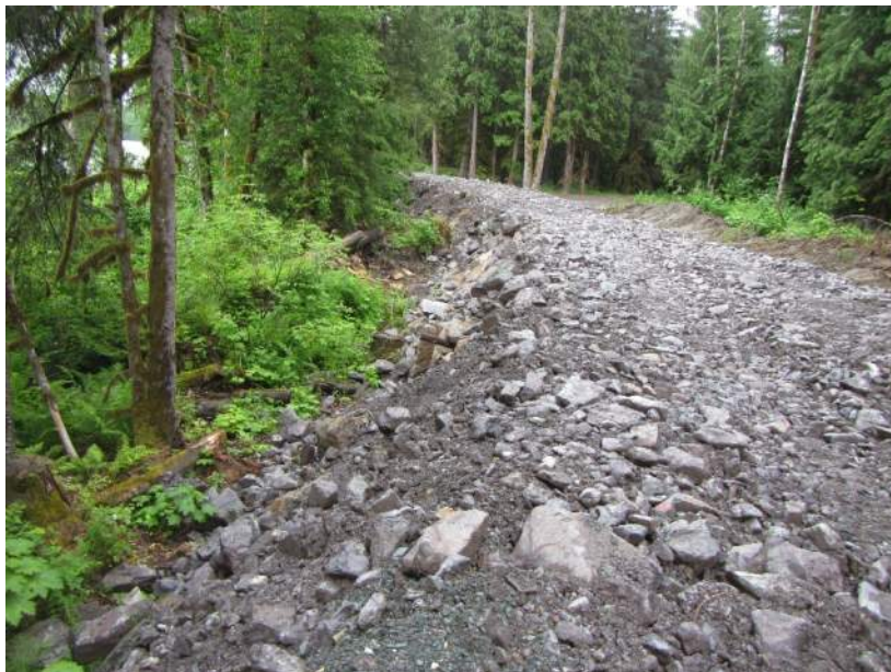
Figure 5.6-2: Existing Riprap Protection– June 21, 2022
