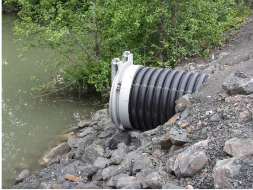
Figure 5.4-2: Existing culvert – June 21, 2022
