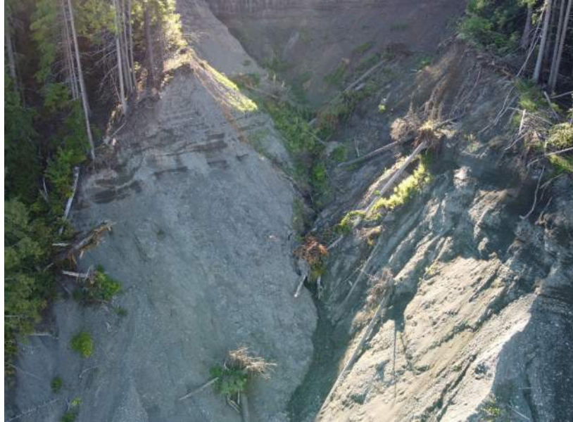
Figure 5.2-1: Toe Stabilization Section – Aug 19, 2022
