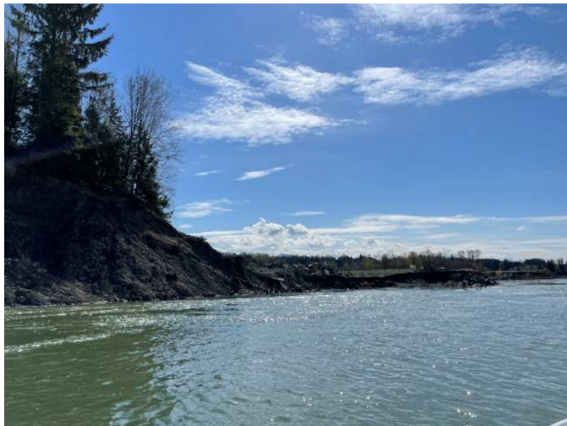
Figure 5.7-2: North end erosion in Dutch Valley – May 13, 2022
