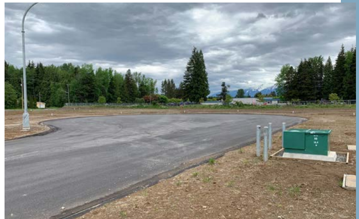
Right: The Nash Drive/Dediluke Place subdivision commenced in 2021 following a subdivision application.
