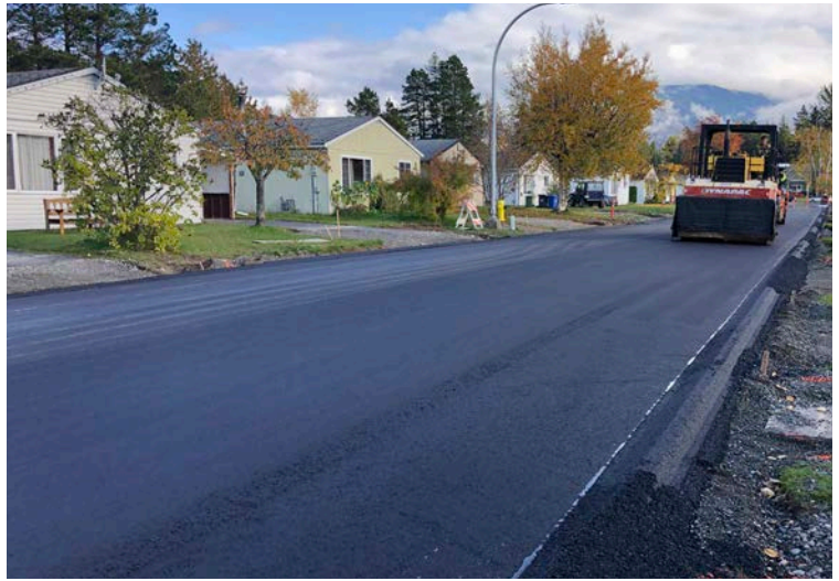
Above: In 2021, Public Works crews completed road reconstruction on Weber Ave. and replaced aging water and storm mains.
