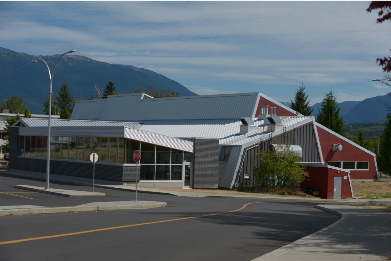
Figure 5: Newly Renovated Terrace & District Aquatic Centre
