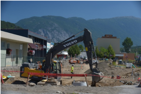
Figure 40: Greig Avenue Reconstruction
