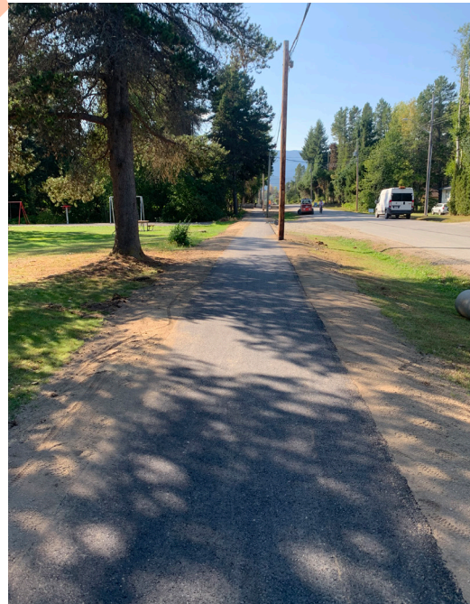
Above: Agar Avenue sidewalk replacement
