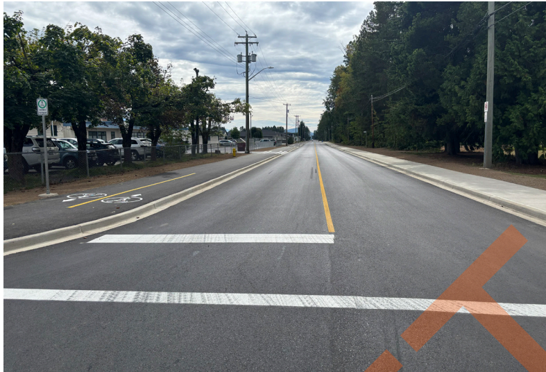
Above: Thomas Street Reconstruction Project
