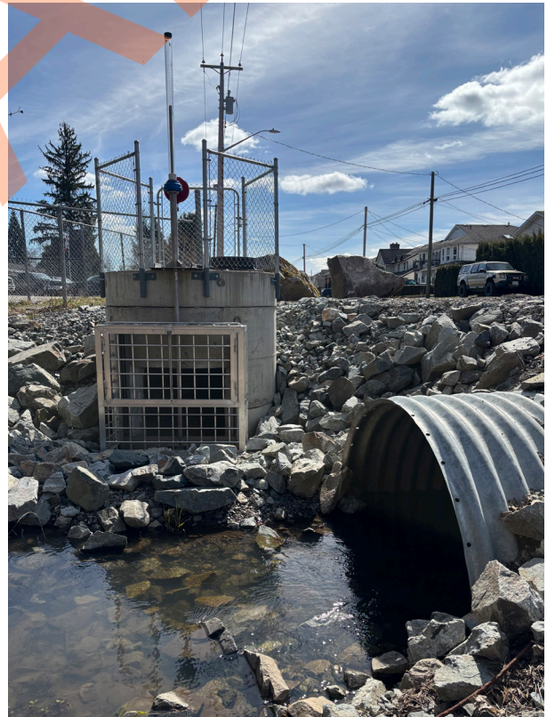
Above: Eby Storm Inlet Repair
