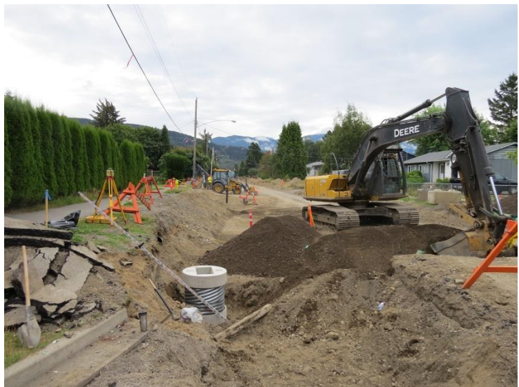
Figure 27: Road reconstruction work
