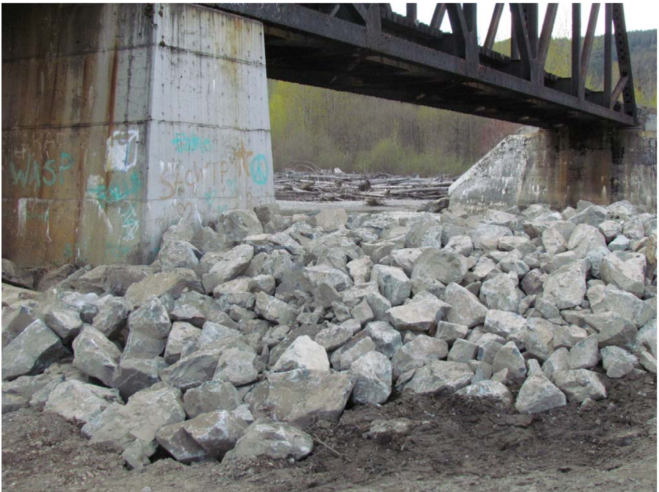
Mitigation Work at Fisherman's Memorial Park
