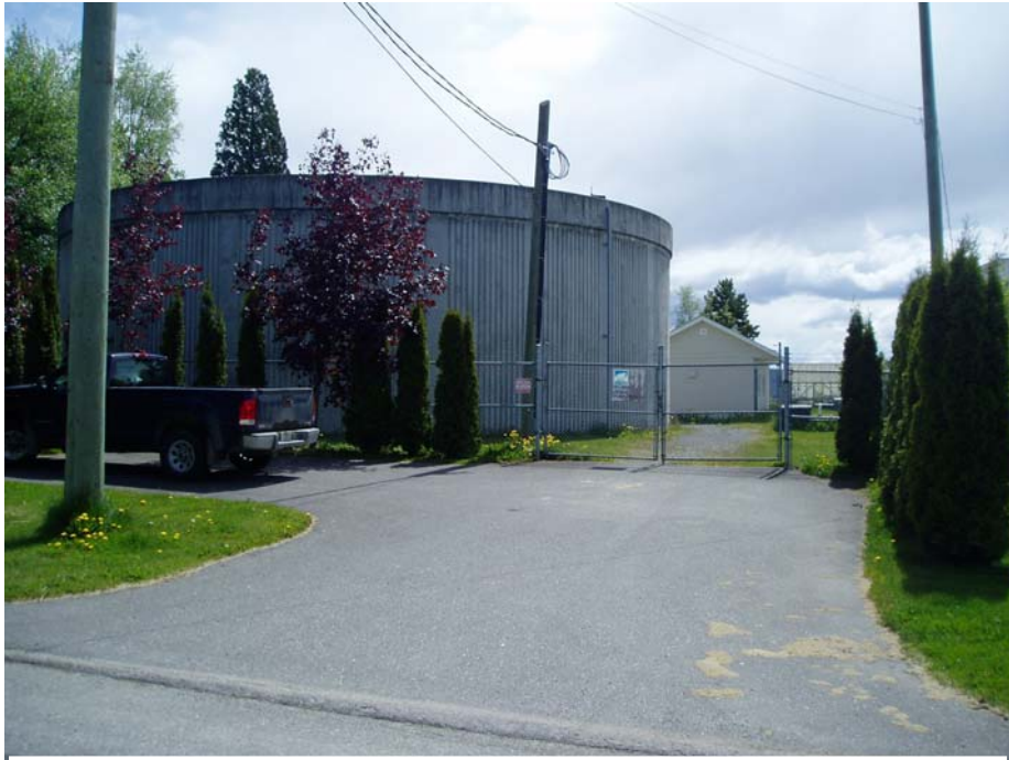
Wilson Street Pump House
