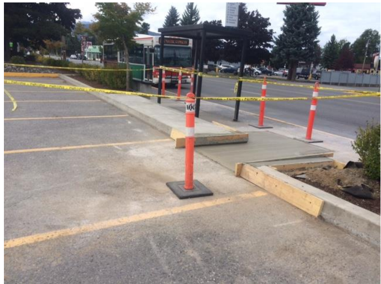
Figure 22: Groundwork for new transit shelter in front of Skeena Mall
