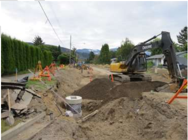
Figure 27: Road reconstruction work
