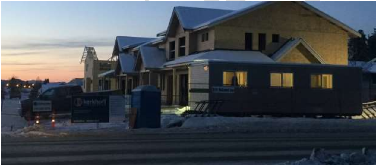
Figure 13: Townhouse development at McConnell Avenue and Cory Drive
