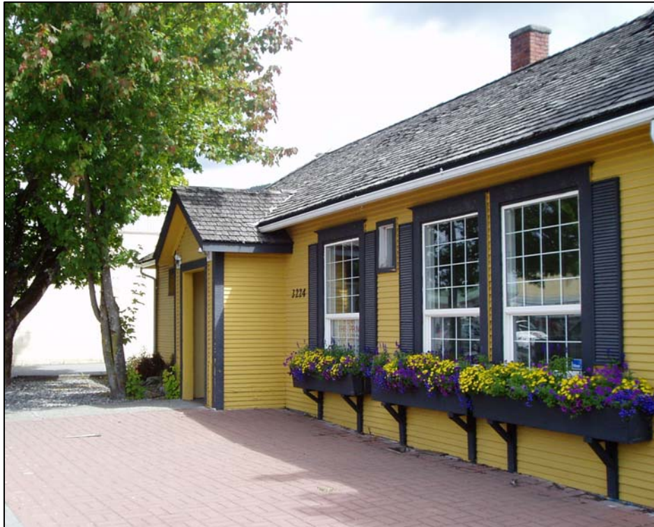
B.C. Provincial Police Building – Kalum Street
